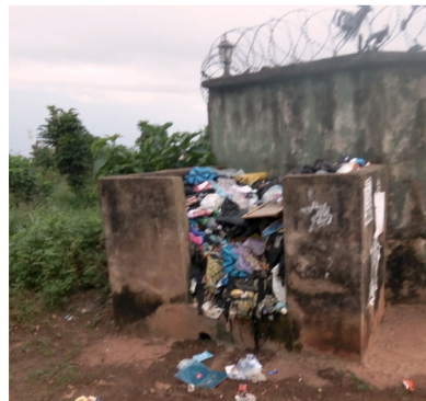
Figure 2e: Fence dumpster
