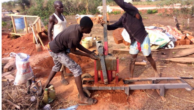
Figure 9: Practical use of machine on building site
