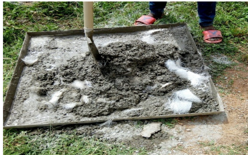
Plate 1: Glass fibres mixed with concrete
