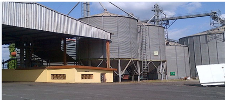
Figure 1: Metal silo storage complex, Akure, Nigeria
