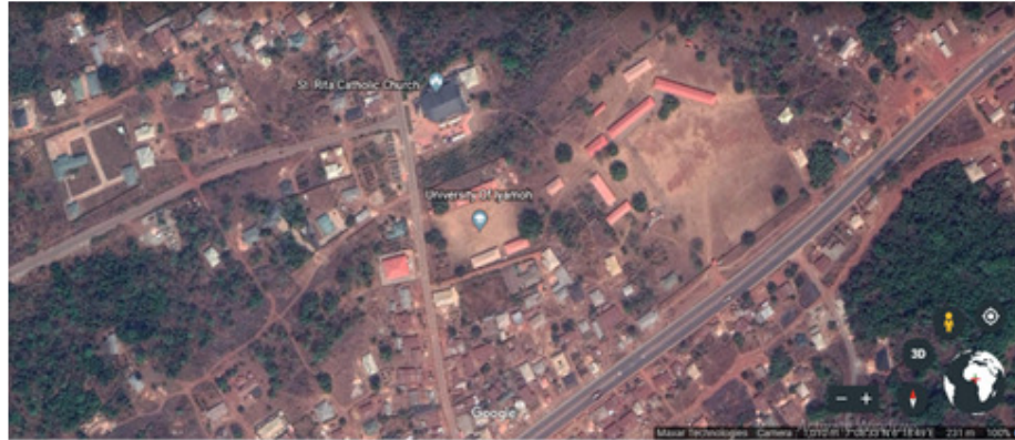
Figure 1: Aerial view of Edo University Iyamho and surrounding community [Source: Google Earth]
