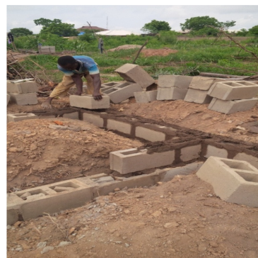
Figure 7: Mason carrying block for laying
