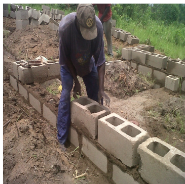
Figure 6: Mason performing block laying
